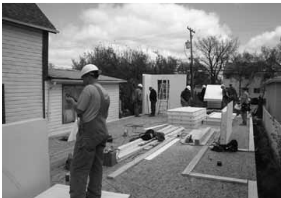
Sentry Homes crew constructs an infill house using SIP panels
