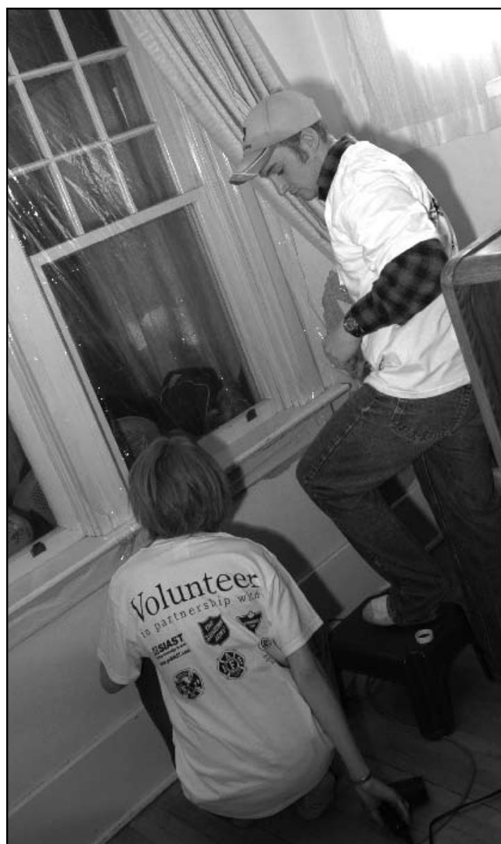
Share the Warmth volunteers seal windows with plastic to trap heat indoors.
